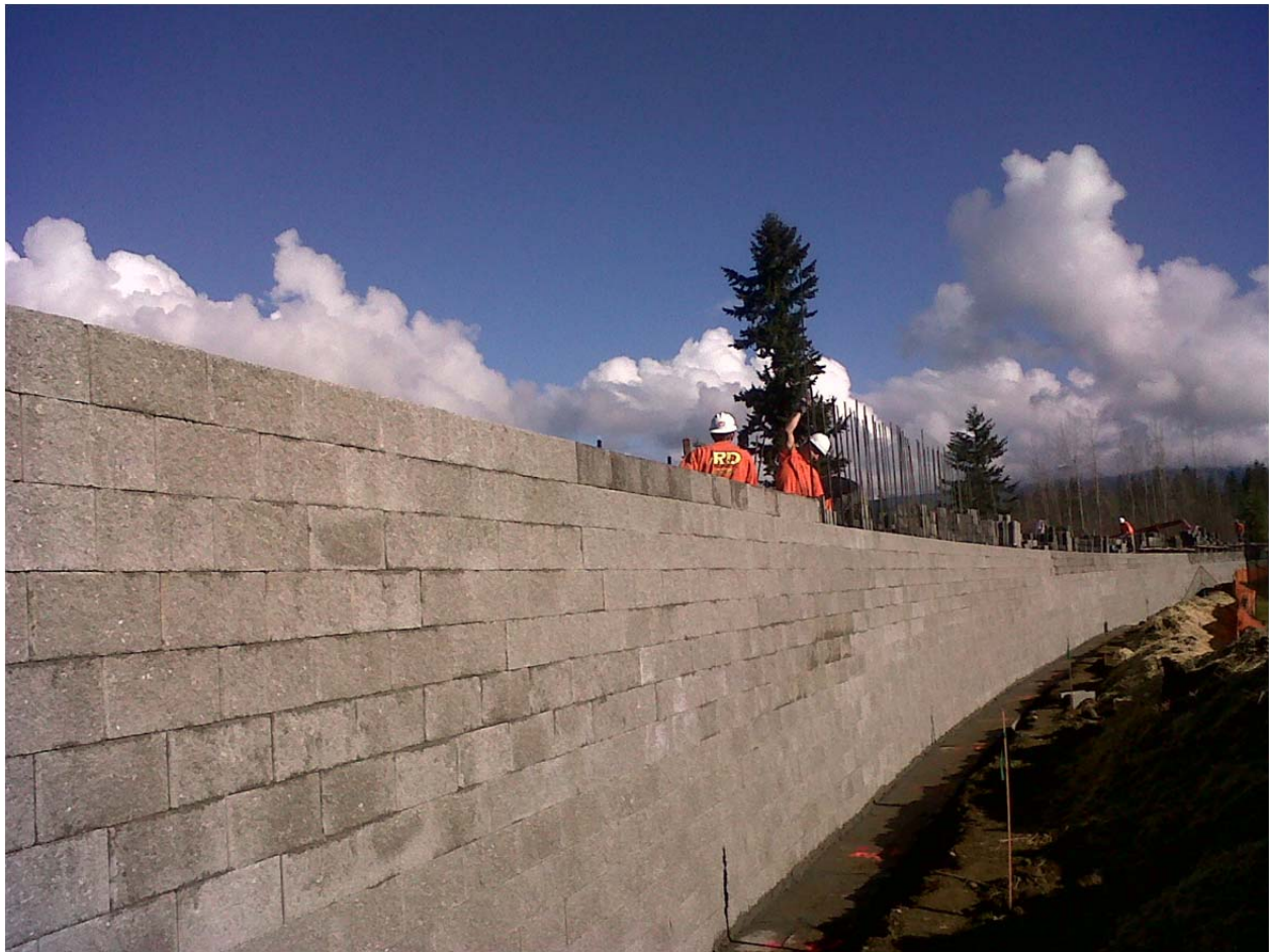
Figure 3: Construction of a CMU wall (courtesy of R&D Masonry, Inc.)
