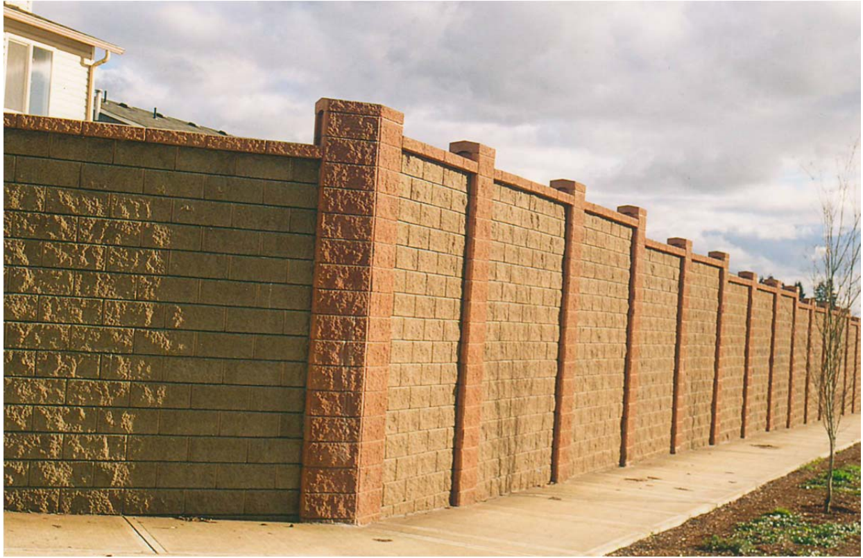
Figure 1: Mortarless CMU sound wall (courtesy of NWCMA)
