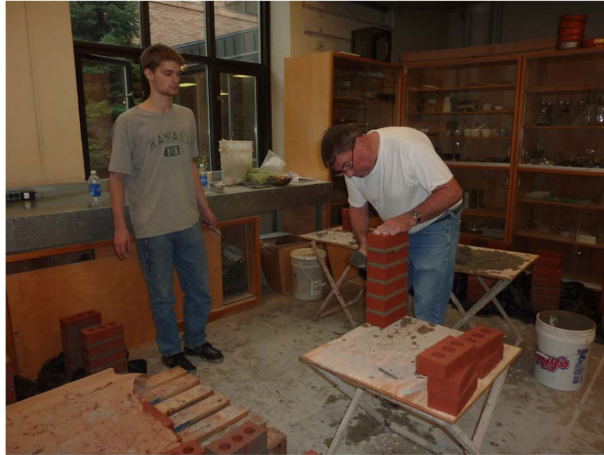
Figure 2: Construction of the Masonry Prisms.
