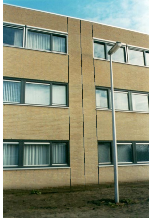
Figure 1: Movement joint in an office building
