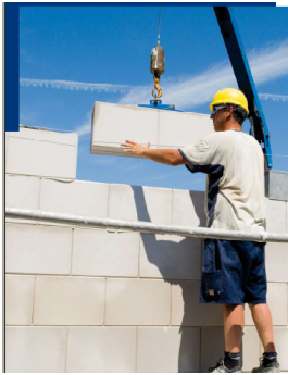
Figure 2 Building with calcium silicate elements and main properties [8], [16].
