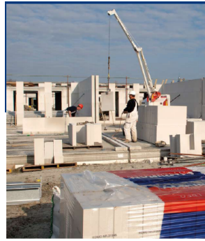
Figure 2 Building with calcium silicate elements and main properties [8], [16].
