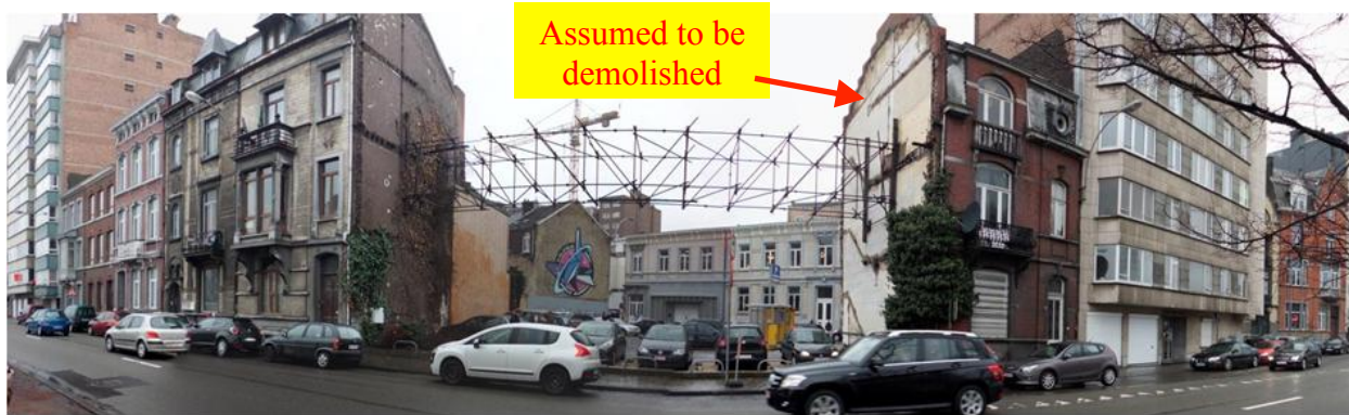
Figure 3 Photograph of the building site taken from river side.
