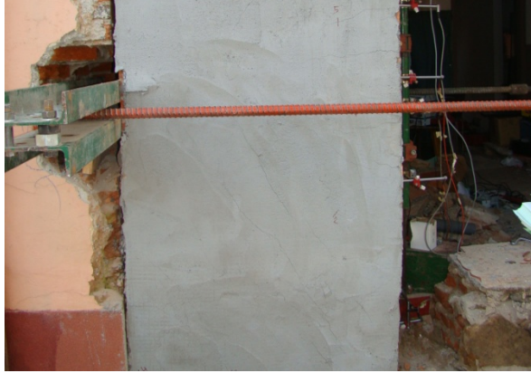
Figure 13: Failure by detachment of GFRP mesh in mortar from the surface
