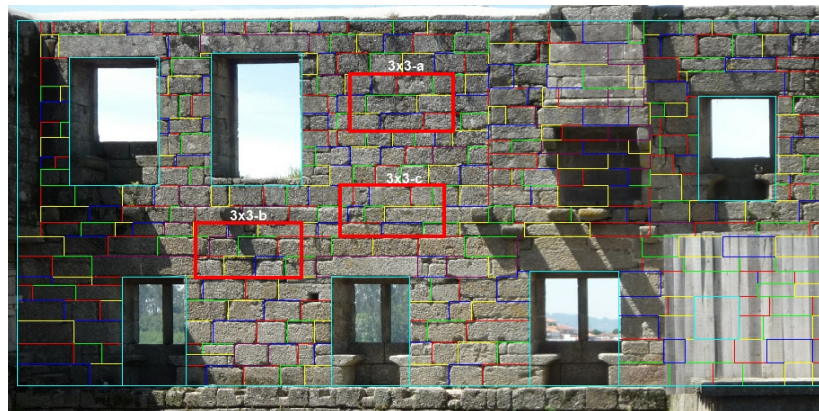
Figure 6: Location of 3x3 Representative Volume Elements (RVEs)
