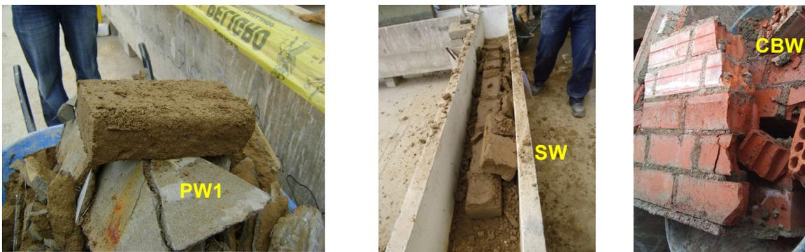
Figure 12: Inspection of masonry units in the base after demolition of the walls.
