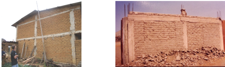
Figure 1: Examples of confined adobe walls in Peru.
