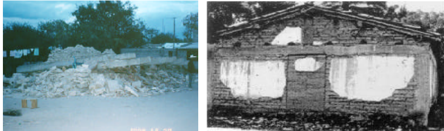
Figure 2: Unreinforced collapsed house (left) and Confined adobe house (right) after the 1995 Omotepec earthquake (EERI, 1995).
