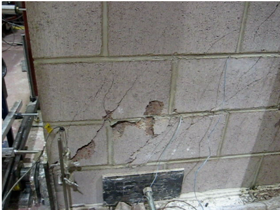
(b) Diagonal cracking with crushing of units at the toe.
