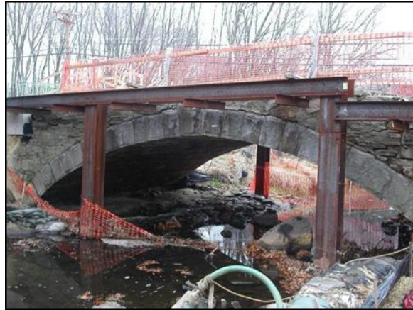
Figure 1: North Masonry Arch with Rehabilitation Auxiliary Framing
