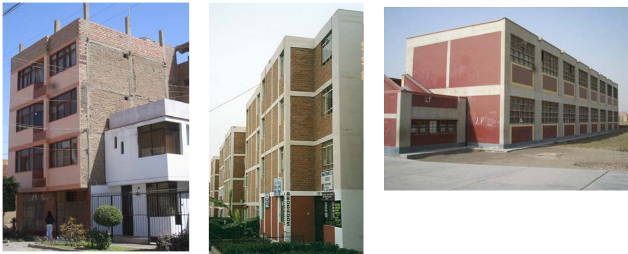
Figure 1: Typical brick masonry loadbearing wall buildings in Peru
