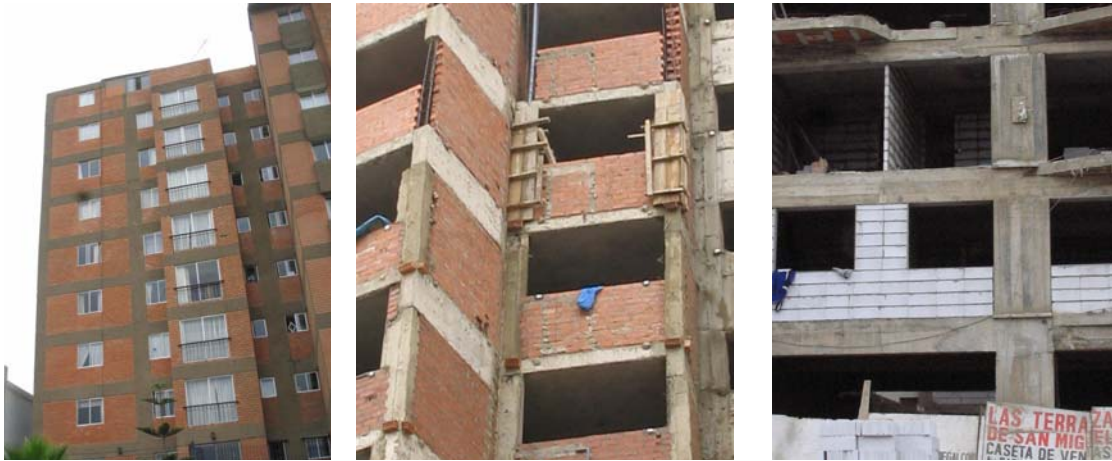
Figure 3: Typical masonry partition walls in Peruvian RC buildings
