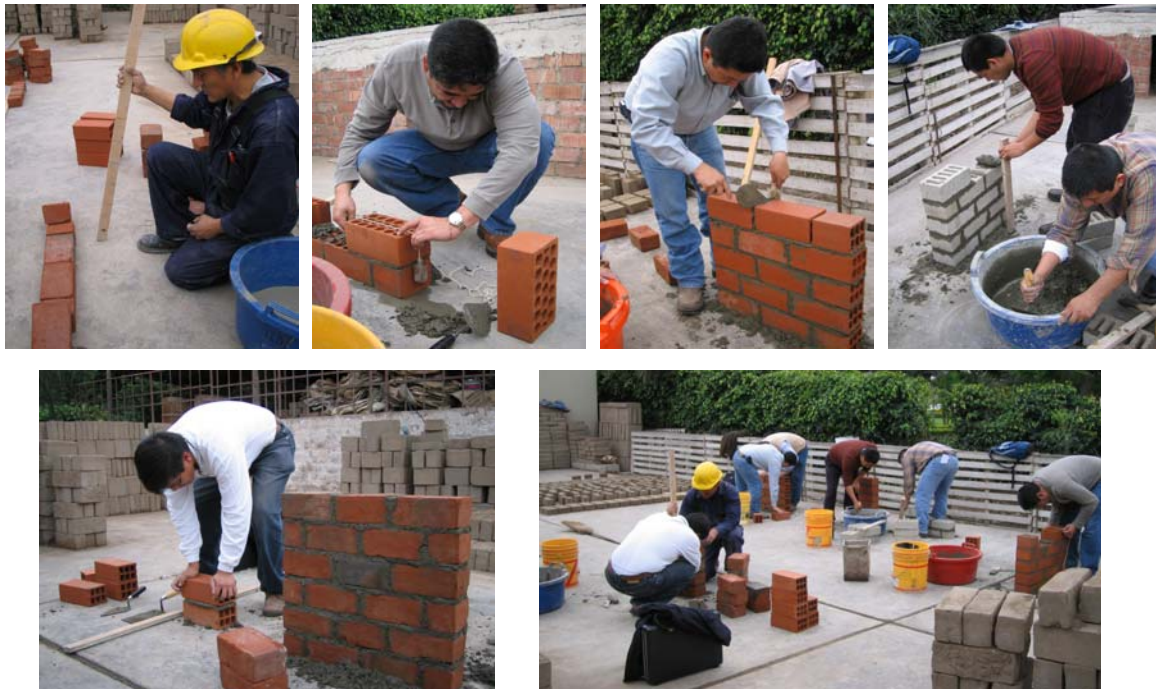
Figure 6: Students performing the construction of prisms and small-size walls specimens
