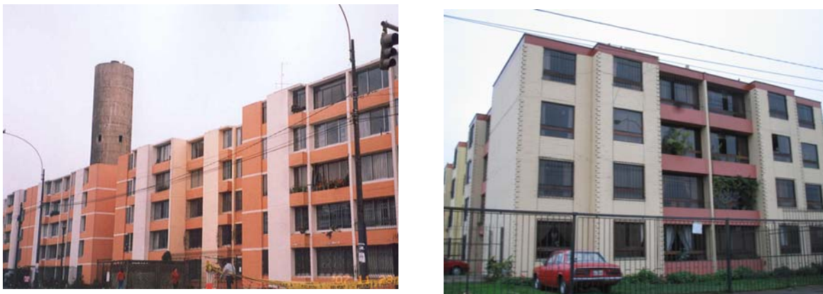
Figure 2: Typical block masonry loadbearing wall buildings in Peru
