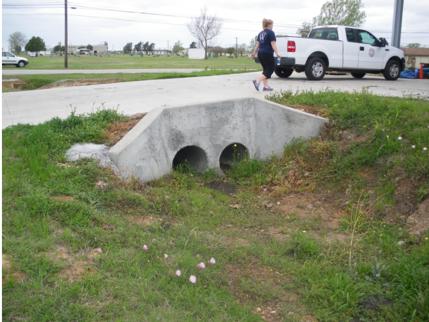
Figure 10: Outlet Headwall located 10 metres downstream of Basin Wall
