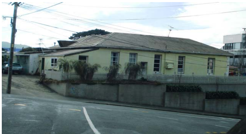
Figure 1: Avon House street view
