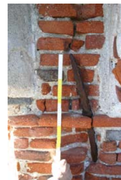
Figure 6: Bolt of a tie rod on the crowning.
