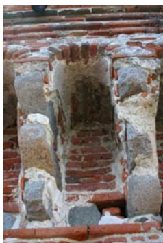
Figure 5: Crowning of the Tower La Marmorata Masserano: details of the damage phenomena.
