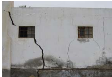
b) Lateral Spreading
