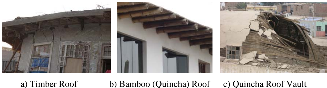
Figure 5: Non-Engineered Roof Systems
