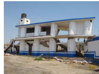
c) Commercial Building
