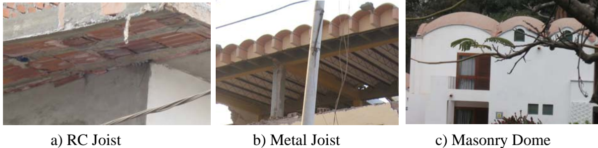
Figure 4: Engineering Floor/Roof Systems
