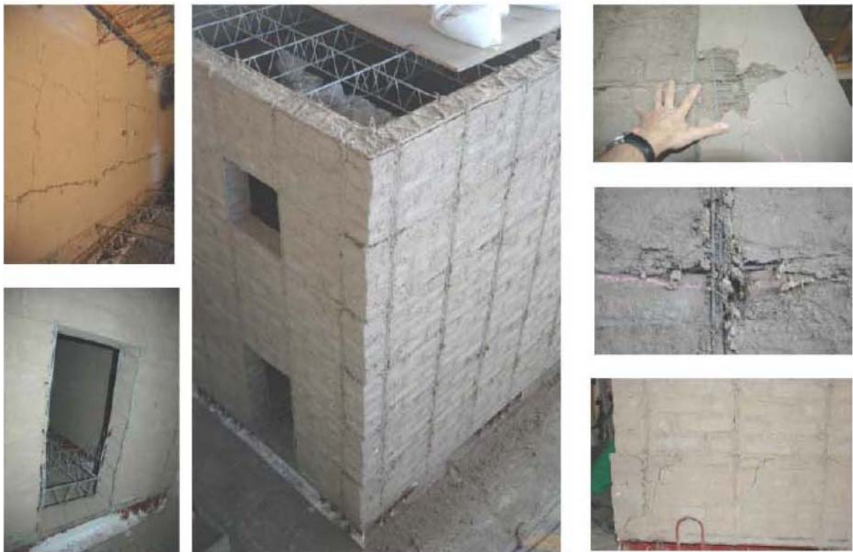
Figure 7: Photographs of damage before 4 th test (130 mm): Left: a) Indoors; b) Entrance. Centre: c) Unrendered sides. Right: d) spalling of render; e) Prefabricated double truss-type reinforcement; f) Cracks in wall.
