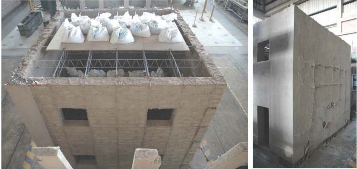
Figure 6: Photographs of cracking after the 4 th test (130 mm): a) Rendered sides; b) unrendered sides
