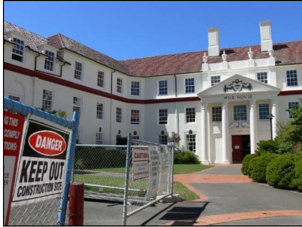
Figure 1: Weir House, case study building (Facing south-east)
