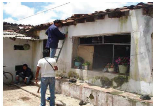
Figure 9: Measurement of vibration in the roof
