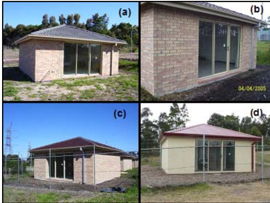
Figure 1: Housing Test Modules (with opening in north wall), (a) Insulated Brick Veneer (b) Insulated Cavity Brick (c) Cavity Brick and (d) Insulated Lightweight
