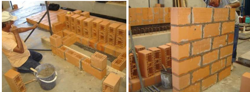
Figure 6: Panel building process 1 – small walls are first built laying blocks vertically
