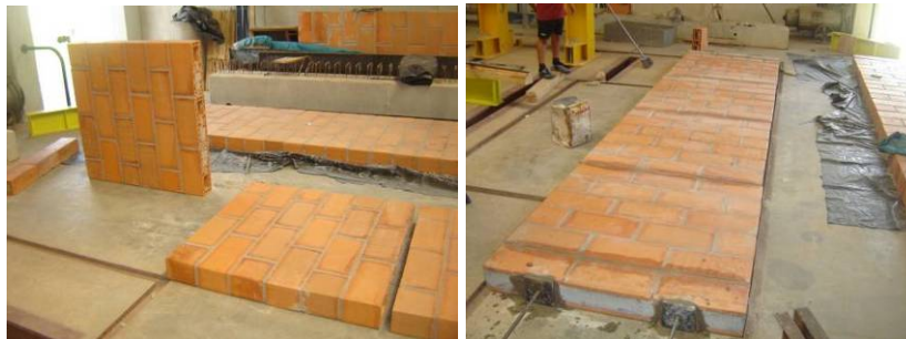
Figure 7: Panel building process 1 – rotate walls and assemble together with prestressing cables
