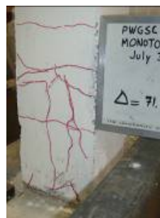
e) Concrete splitting at the Tension column Drift 3.55%
