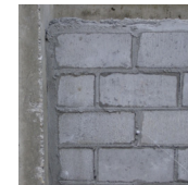
Mortar joints
