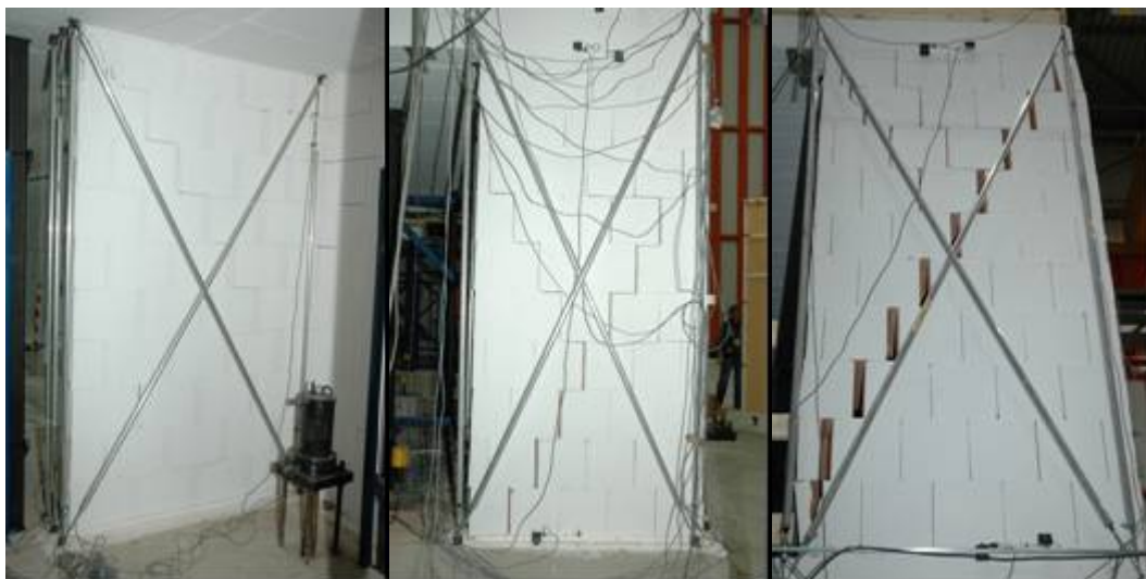
Figure 9: Crack pattern of shear walls after the test with ground acceleration 0,22 g; main shear wall ground floor (left), external wall ground floor (centre) and external wall first floor (right)
