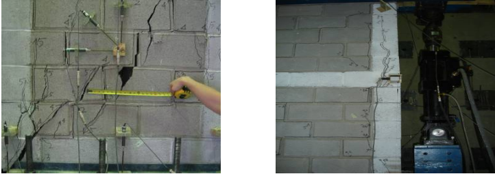
Figure 5: Cracking and Failure mode of partially grouted walls [9]
