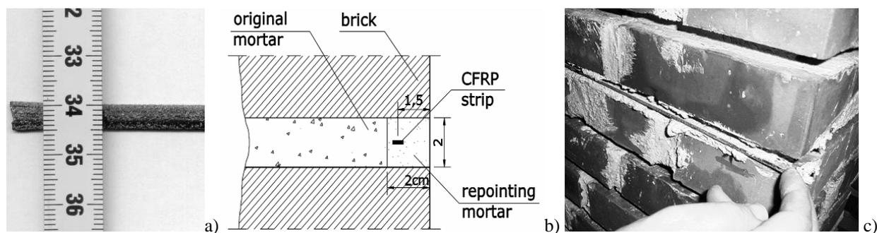
**Figure 1: Bed joints reinforcement technique: a) CFRP thin strip, b) reinforcement positioning detail, c) insertion of a CFRP thin strip in a masonry panel**
