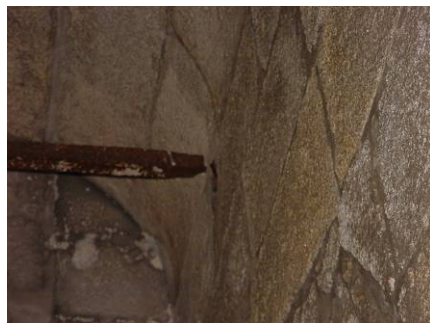
Figure 9: Ancient Tower Ties: (a) Deformed Anchorage ( T_1 ); (b) Details of Broken Tie ( T_3 ).
