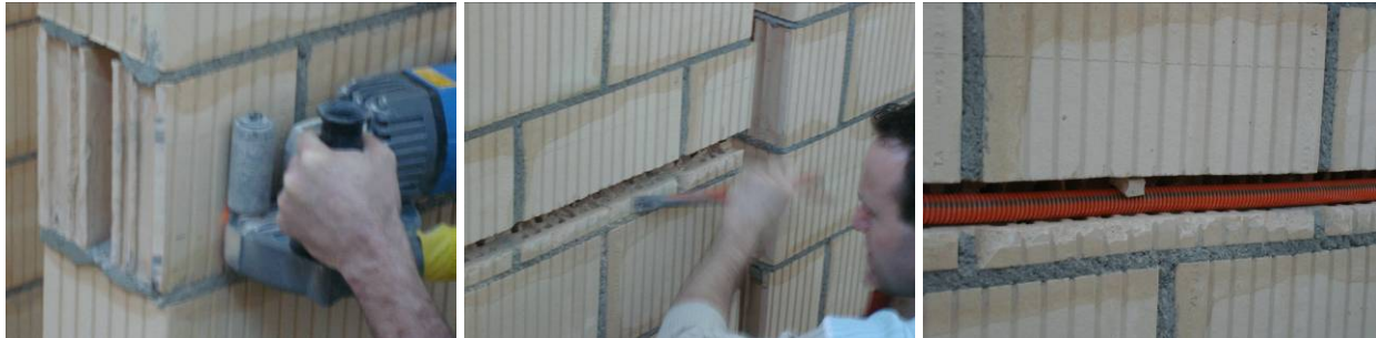
Figure 3: Preparation of the Specimen with Horizontal Chase
