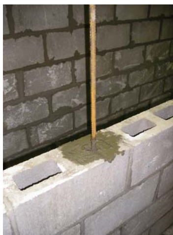
Figure 3: Grouting of core with reinforcement after four courses had been laid.
