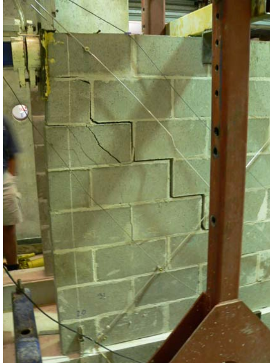
Figure 10: Actual cracking from the loading point (top left of the wall in this view) in wall 2 (1.6 m spaced reinforcement).
