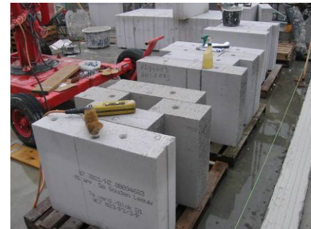
Figure 4: CASIELs on site
