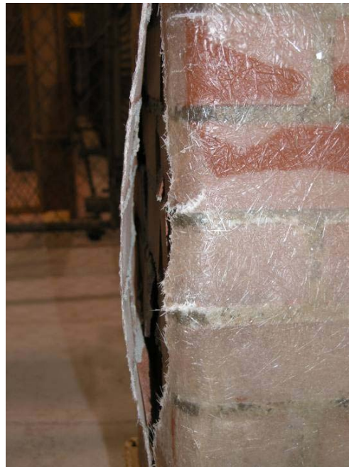
Figure 7 –Failure of SGFRP laminate in AP2 (above) showing a mix of Mode I and Mode III cracking and BP4 (below) showing only Mode III
