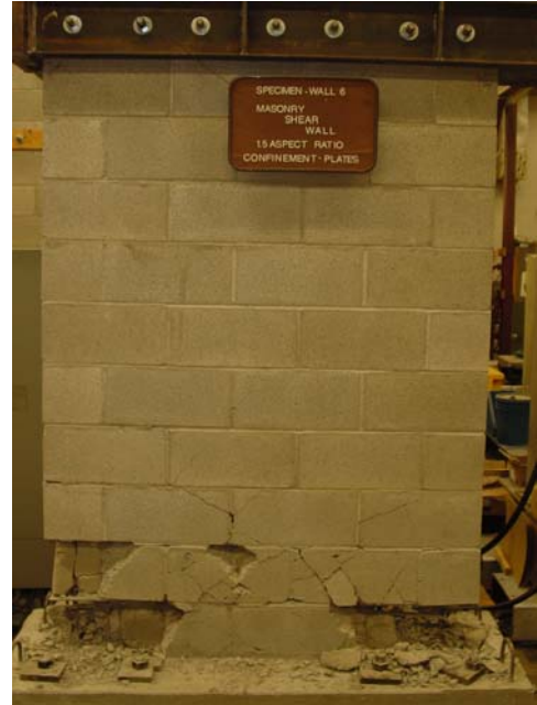
Figure 6 -Wall 6 After Testing
