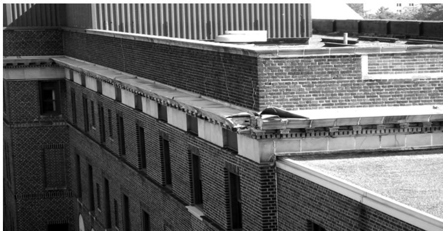
Figure 5 – South Building cornice, southwest corner
