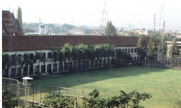
Figure 2 - Suankularb Building before Renovation
