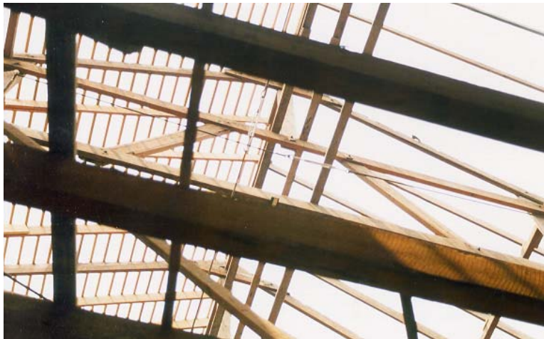
Figure 6 - Roof under Construction
