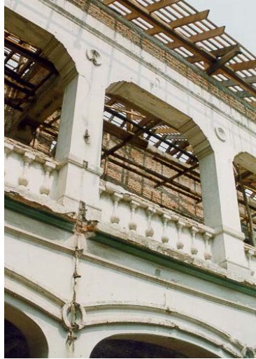
Figure 7 -Existing Arches and Moldings
