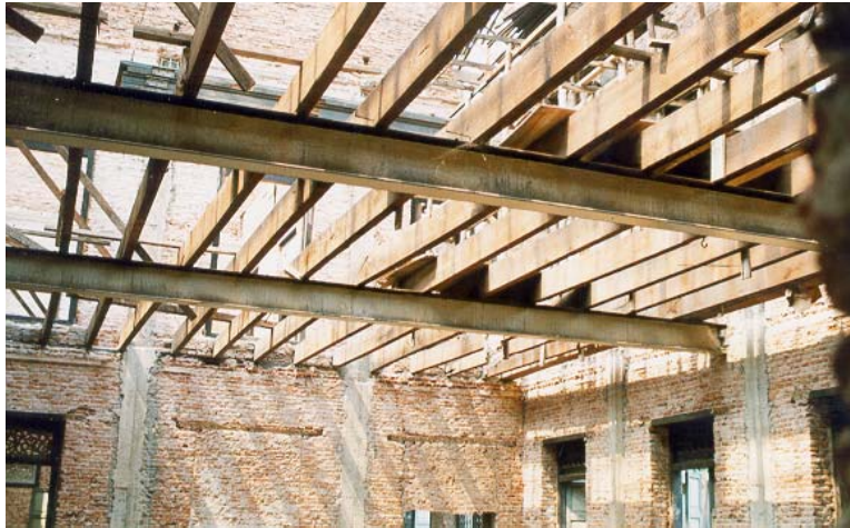
Figure 8 - Original Structure of Second Floor
