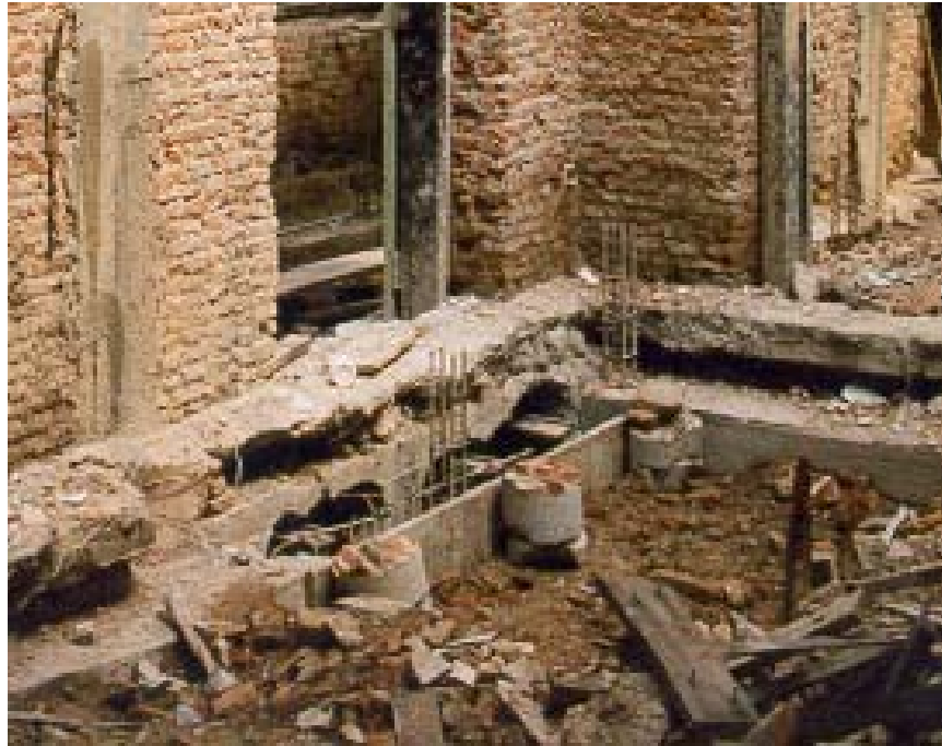
Figure 9 - Micro-piles, New Ground Beams, and Coring of Existing Grade Beam
