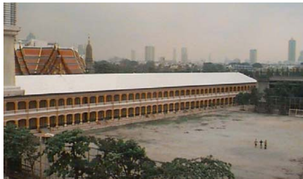
Figure 3 - Suankularb Building after Renovation
