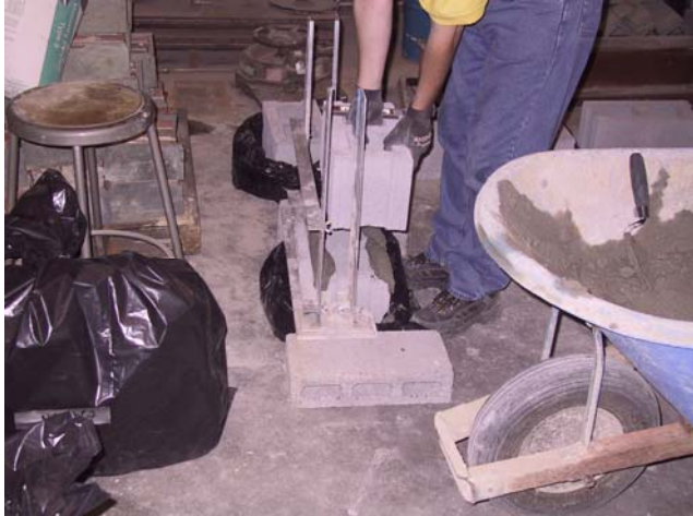
Figure 1 - Lower Block Buttered with Mortar
