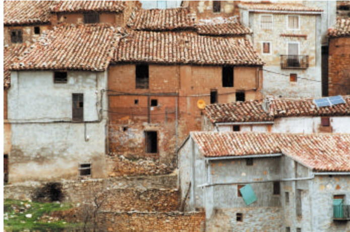
Figure 5 - View of the House Chosen for the Pilot Restoration Project
