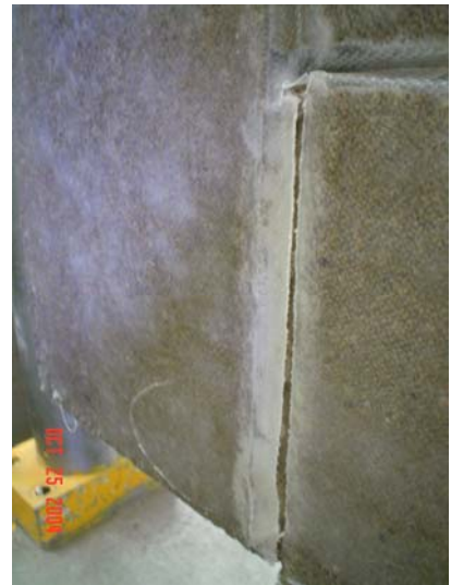
Figure 6 – GFRP Failure
