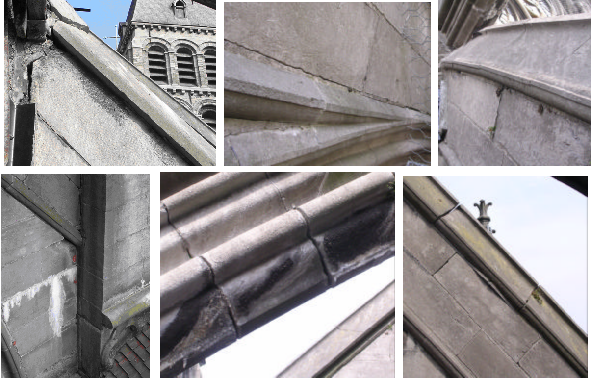
Figure 9 - Actual configuration: several views of flying-buttresses
