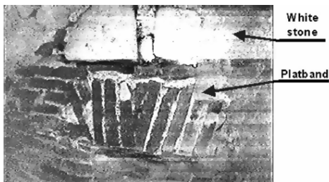
Figure 12 – Pisece Castle. Videoboroscopes and detail of the masonry in the position POS1
