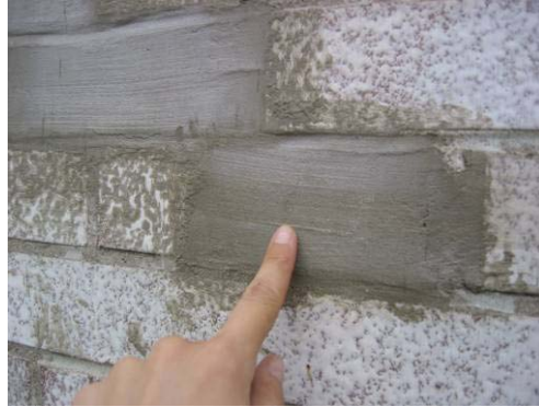
Figure 3 – ‘Parge’ Repair of Spalled Brick
