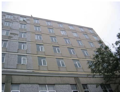
Figure 5 – Work Proceeding on West Elevation
