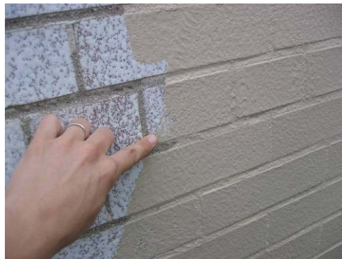
Figure 4 – Application of Elastomeric Silicone Coating
