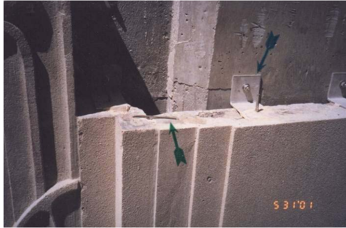
Figure 12 – Reinstalled Stone with New Stainless Steel Supports
