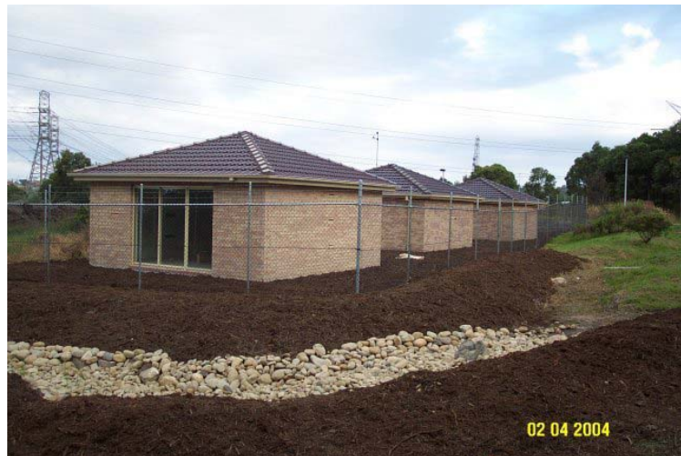
Figure 1 – The Three Building Modules for Thermal Testing.
