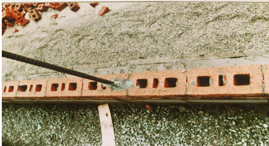
Figure 3 – Reinforced Hollow Clay Brick
