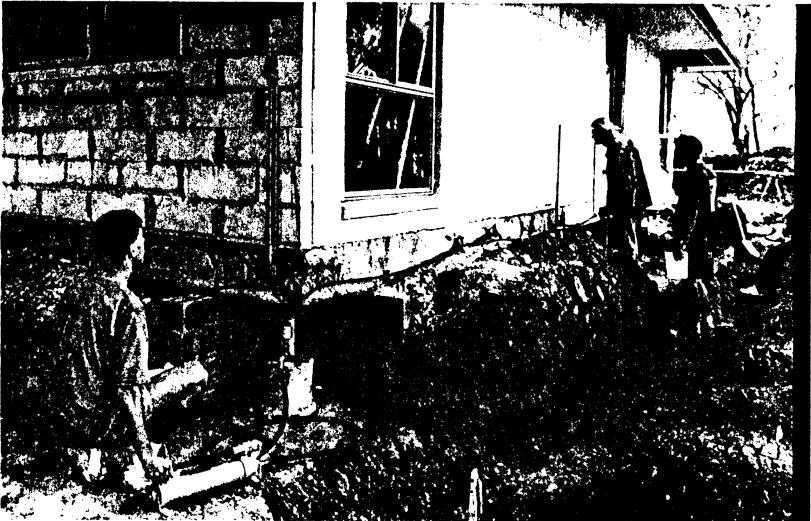
Figure 4. Typical Jacking Location
