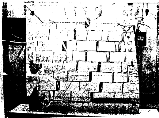
(b) Racking Test
