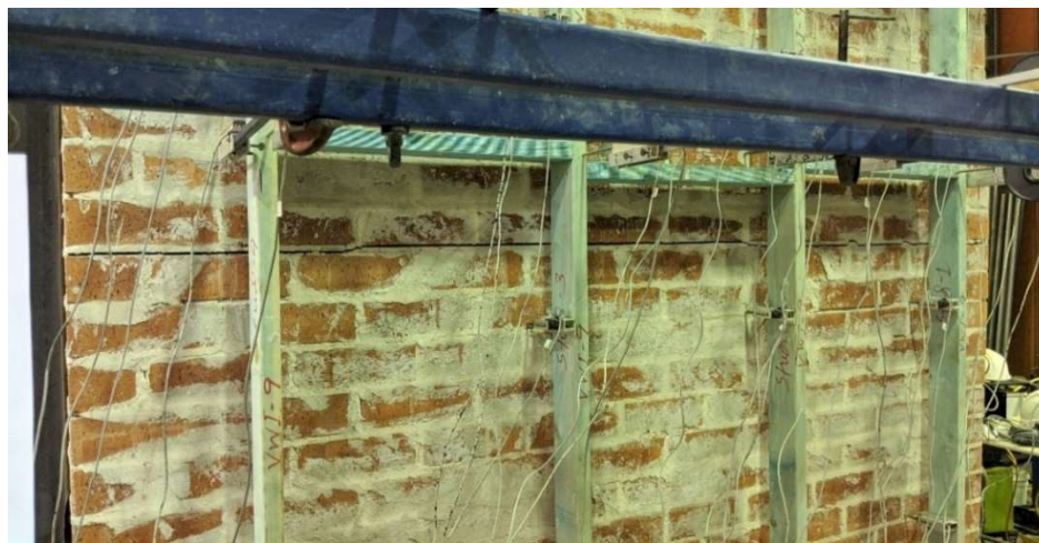
Figure 8: Brick Veneer Cracking Under Out-of-plane Loading
