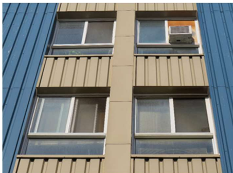
Figure 6: St. Clair Birchmount I. Metal rainscreen assembly in front of existing brick veneer.
