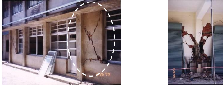
Figure 1: Common types of CM wing-walls in Taiwan: a) Single Wing-Wall; b) Twin Wing-Wall
