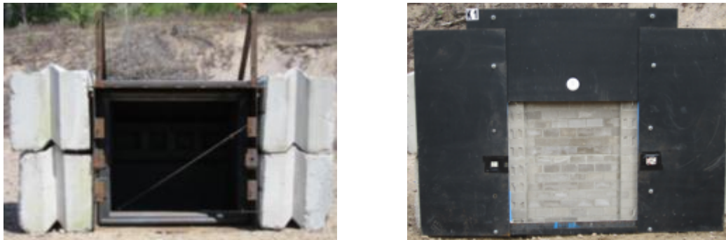
Figure 3: Test frame: a) The reaction frame without wing-walls, b) Wing-walls attached and wall loaded
