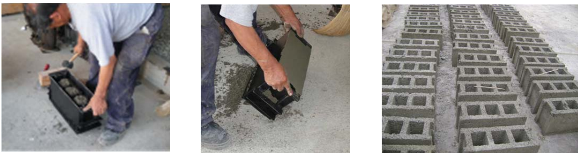
Figure 2: CMU preparation: a) Metallic form; b) Solid surface; c) Drying
