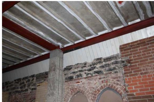
Figure 11: Floor-to-Wall Connection
