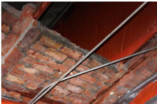
Figure 10: Terracotta Attic Floor
