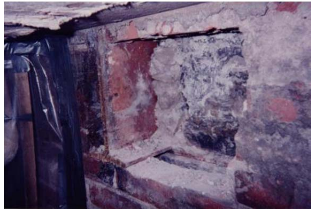
Figure 9: An Original Beam Bearing Detail
