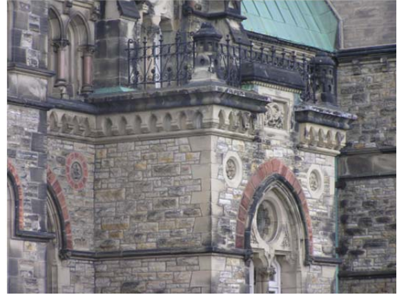
Figure 3: Typical Exterior Walls
