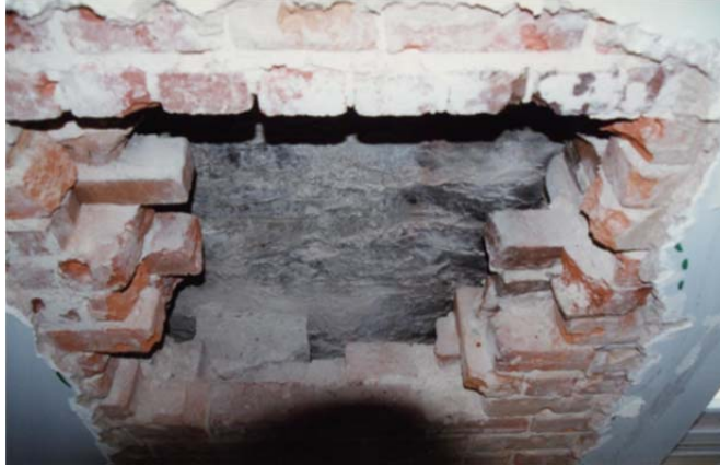
Figure 2: Typical Cavity Wall
