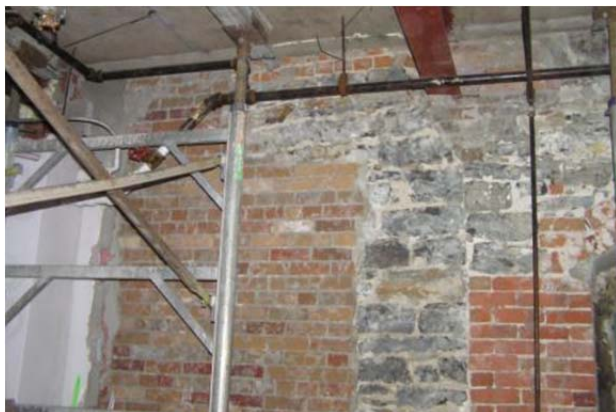
Figure 4: Brick and Stone Masonry Wall
