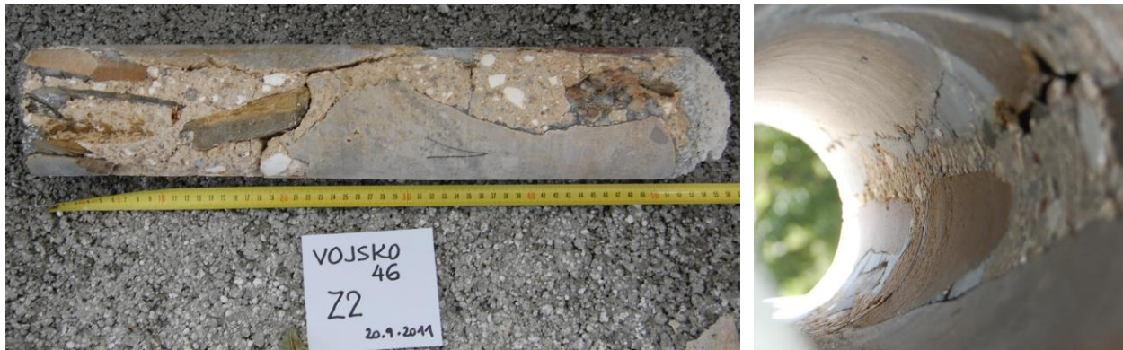
Figure 4: Very effective grouting - the grout has filled the voids and connected together the stones and mortar
