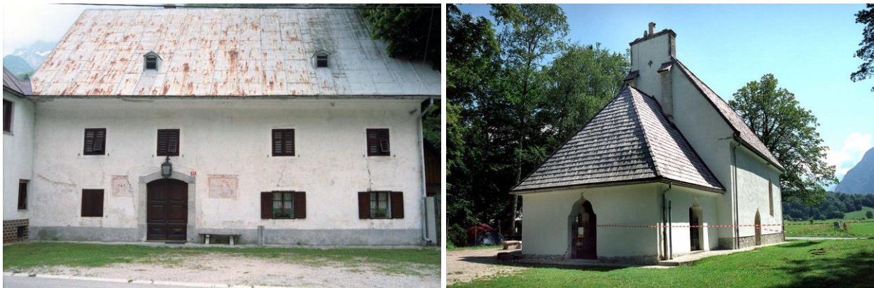
Figure 1: a) Original stone-masonry building; b) Stone-masonry church in Bovec – the upper part of the bell wall overturned due to out-of-plane vibrations
