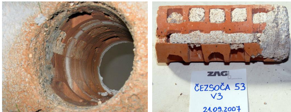
Figure 5: A retrofitted brick masonry wall: a) the surface of the borehole, b) the core
