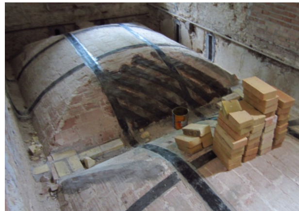
Figure 15: Hardwire and C-FRP repair and strengthening of vaults
