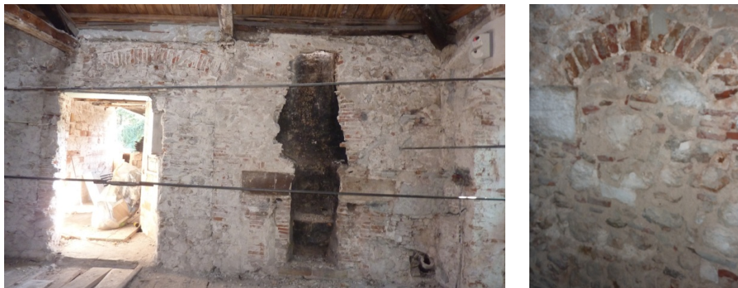
Figure 5: View of chaotic wall organization with flues and heterogeneity of texture
