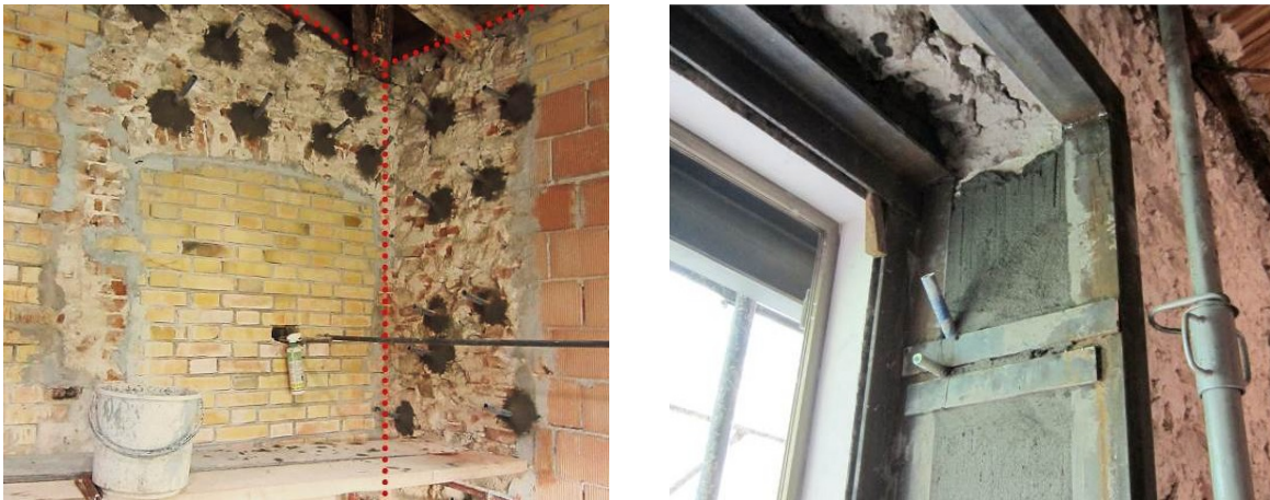
Figure 13: Injections, brick texturing and frame stiffening around windows
