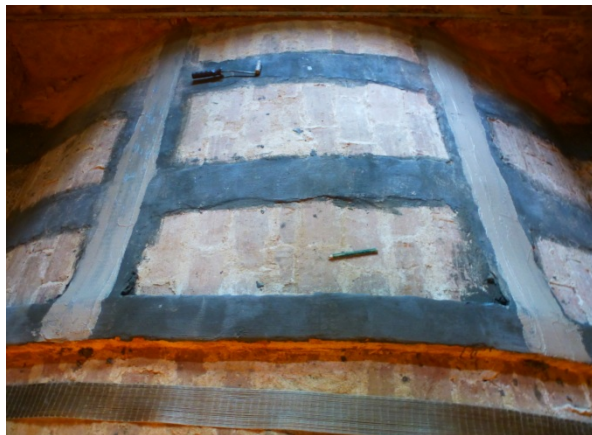
Figure 15: Hardwire and C-FRP repair and strengthening of vaults
