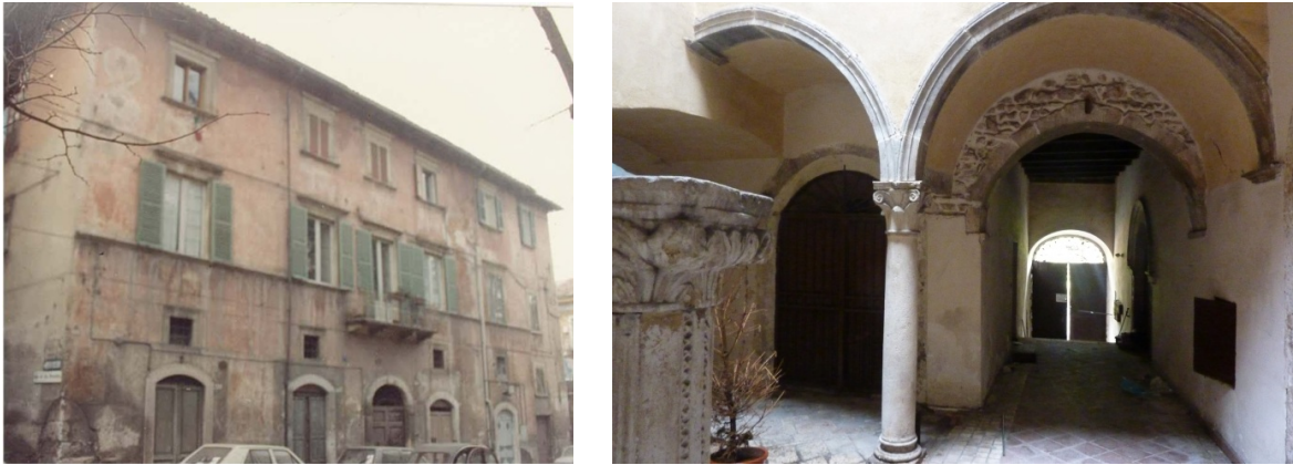
Figure 1: View of Micheletti Palace and open internal court
